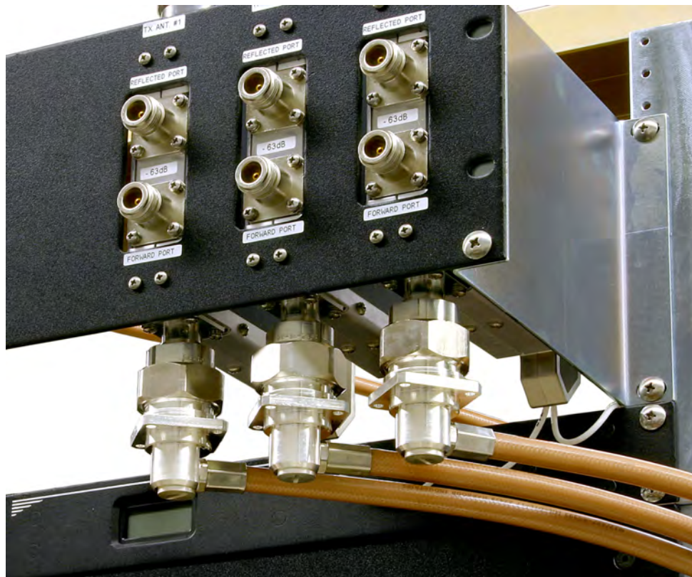
Figure 3: Combiner outputs connect to the ACM inputs.
